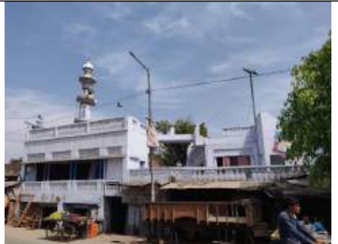
A view of Mosque along the project road
