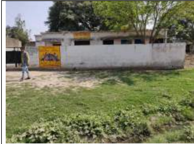
A view of School along the project road
