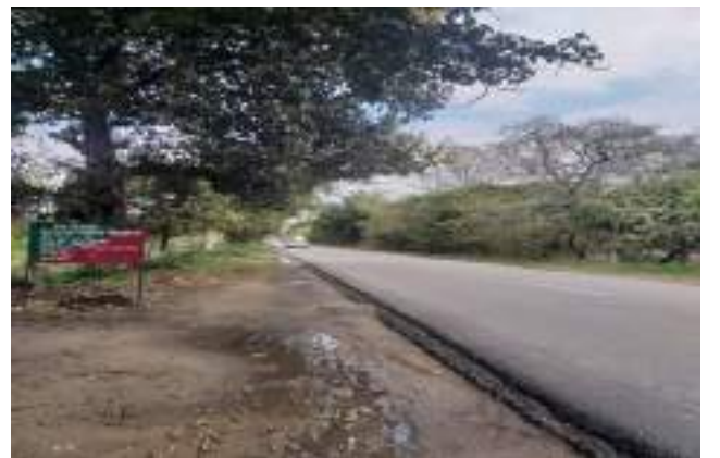
A view of project road at Shahjahanpur
