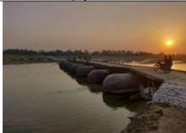
A view of Pipa Bridge to be impacted along the project road at Shahjahanpur
