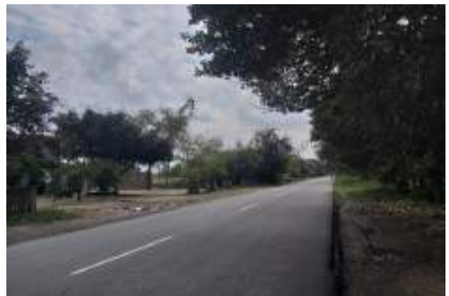
A view of project road at Shahjahanpur
